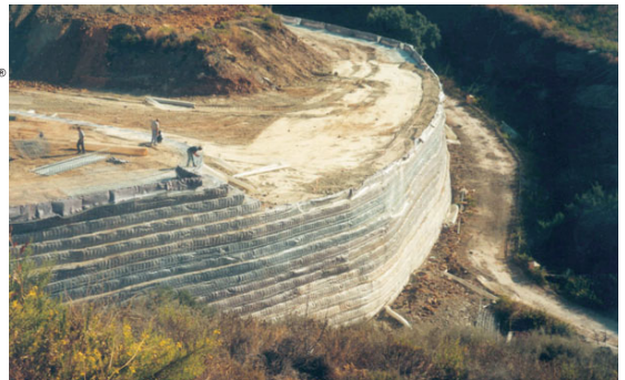
Mechanically stabilised earth (MSE) wall construction
