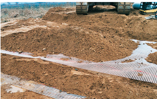
Two layers of Ariankhak Iranian Group® a road dam reinforcement
