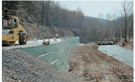
Railroad slope stabilisation
