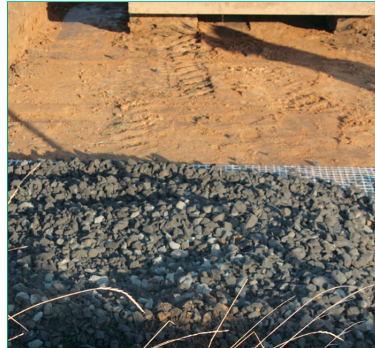
Fig. 17 Placement of base course gravel over the GEOGRID section
