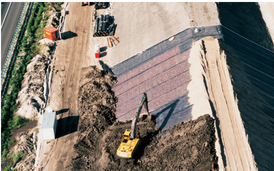
Slope reinforcement of a noise barrier with Ariankhak Iranian Group®
